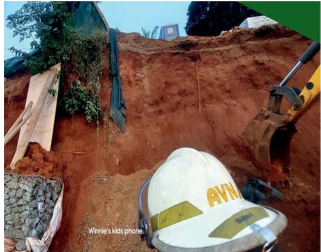
A sand bank collapsed while builders were working on site, covering five (5) construction workers.
