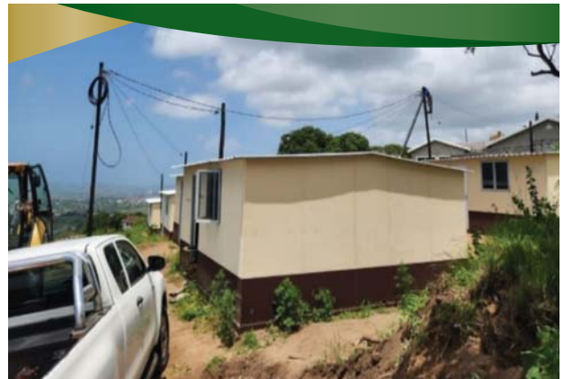
Temporary Residential Units (TRU's) electrified.
