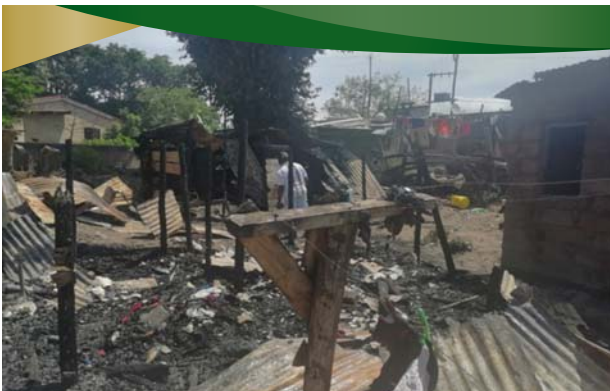
Aftermath following a structural fire incident in Ward 04 (Shakashead) during the month of October 2022
