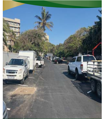
Upgrade to Willard Beach Car Park
