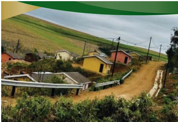
Steve Biko housing electrification completed.
