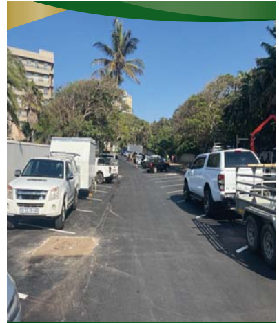
Upgrade to Willard Beach Car Park
