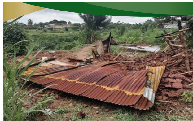
Aftermath following a structural fire incident in Ward 27 (Madundube) during the month of December 2022
