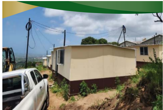
Temporary Residential Units (TRU's) electrified.
